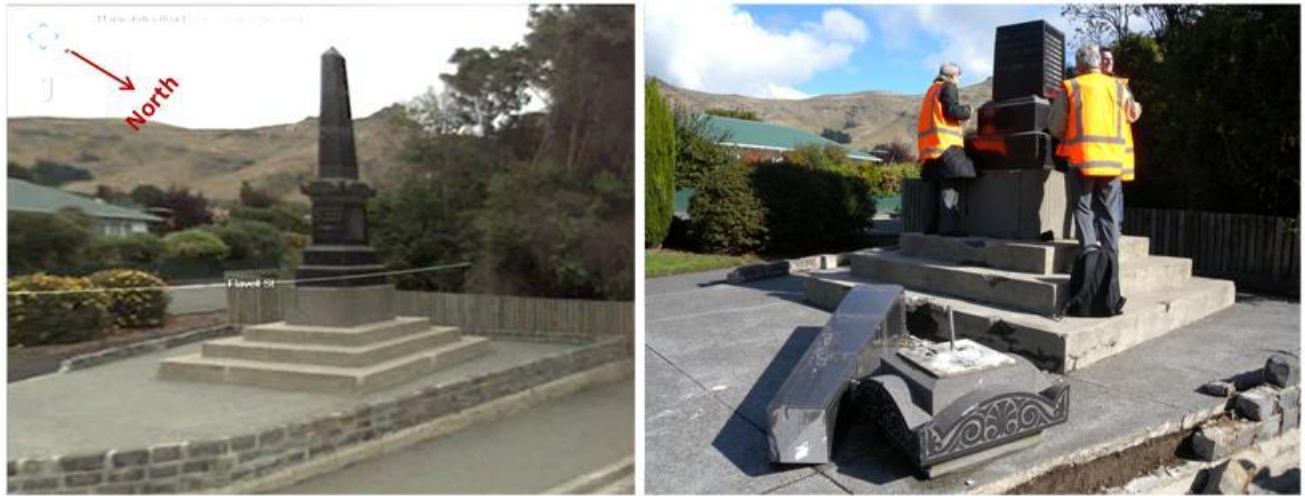
Figure 2.54. Obelisk at the corner of Bridle Path Road and Martindales Road close to HVSC station before Christchurch earthquake (left). Fallen obelisk after the earthquake (right).
