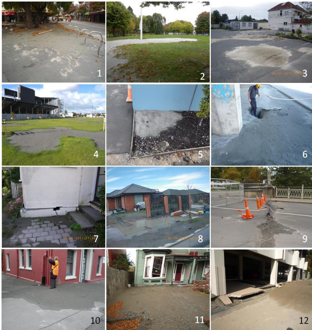
Figure 2.62. Photos of liquefied sites after Christchurch earthquake.
