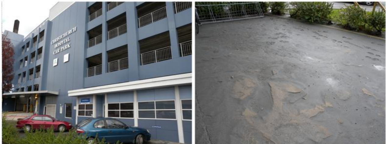
Figure 2.17. Christchurch Hospital Car Park (239 Antigua St) adjacent to CHHC seismic station building (left). Ejected sand in front of Christchurch Hospital Car Park 40 days after the earthquake (right).
