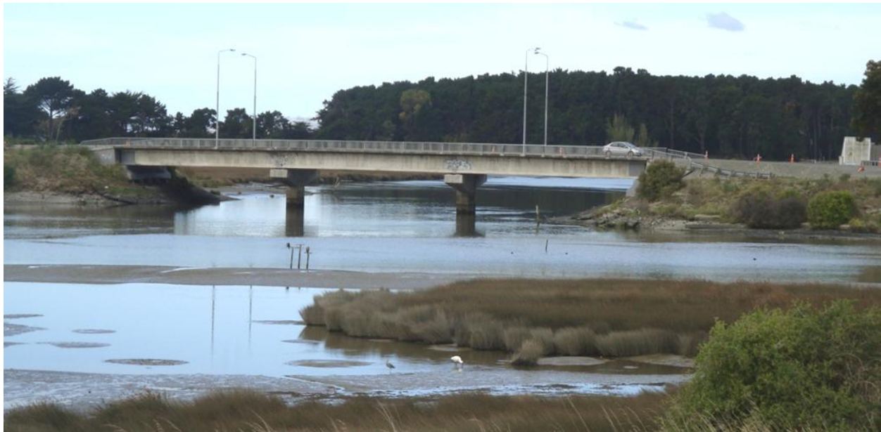
Figure 4.31. South Bridge Road Bridge (B8 on map of Figure 4.1) after Christchurch earthquake.
