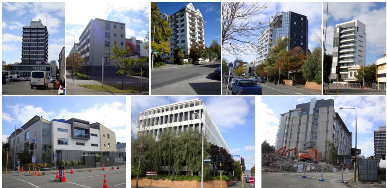
Figure 3.56. Modern RC buildings performing satisfactorily.
