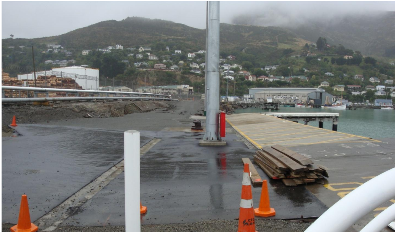
Figure 5.23. Large settlement of the backfill (site W3 in the map of Figure 5.6).
