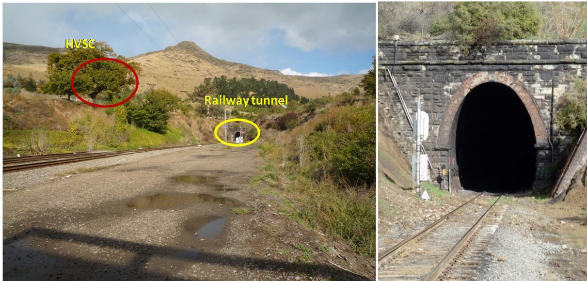
Figure 2.48. The excavation adjacent to HVSC station, leading to railway tunnel. The remnants of rain water show that it cannot be easily absorbed by the soil which is indicative of clayey soil with low permeability(left). The entrance to the railway tunnel. No damage was reported (right).
