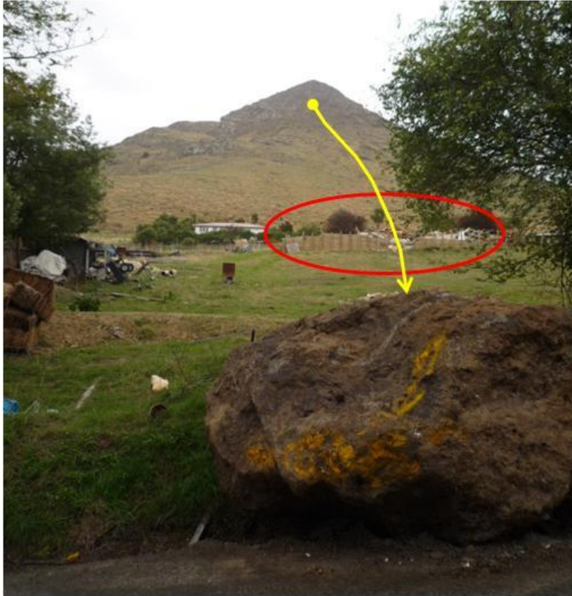
Figure 5.2. Boulder struck through a house at 241 Governors Bay Road in Rapaki (site S1 in the map of Figure 5.1).
