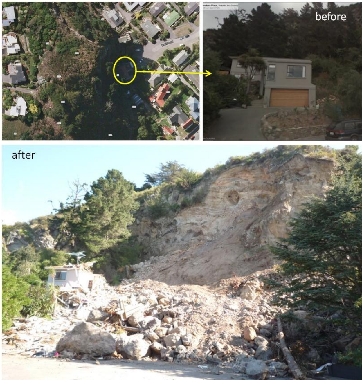
Figure 5.3. House collapsed by rock fall at Reakura Pl. in Redcliffs (site S2 in the map of Figure 5.1).
