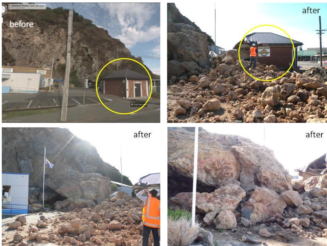
Figure 5.5. Extensive rock fall behind the RSA building at 34 Wakefield Ave, in Sumner (site S4 in the map of Figure 5.1).
