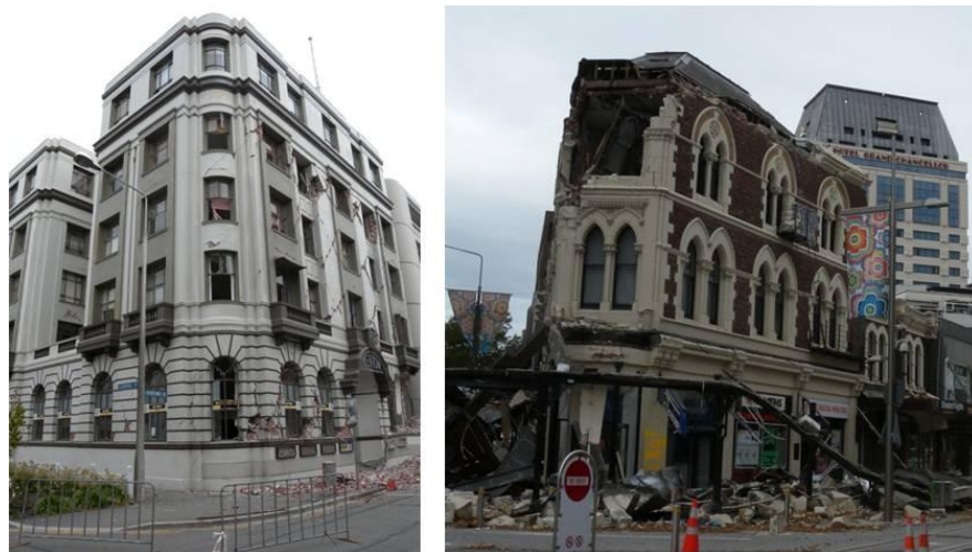
Figure 3.17. Severely damaged building at Hereford St with characteristic shear cracks and historical building at Stewart Square.
