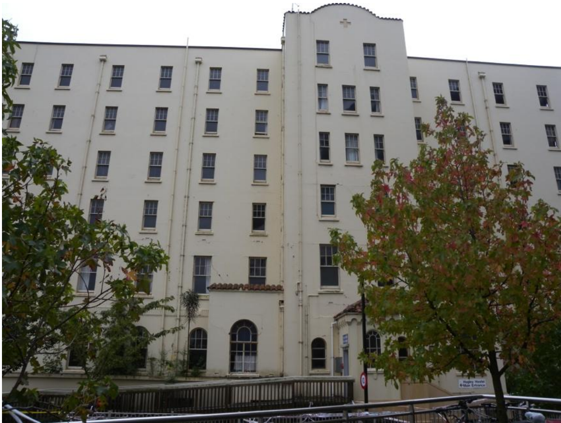
Figure 3.41. The old unreinforced masonry block for nurses, that has moderately damaged during the earthquake.
