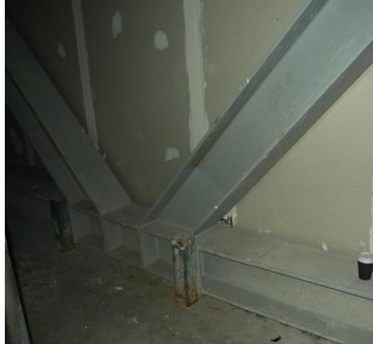
Figure 3.40. Eccentrically placed steel bracing in the superstructure of the Women's Hospital.
