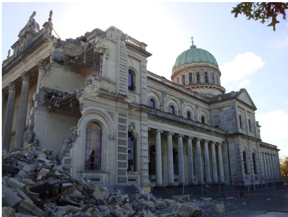
Figure 2.23. Partial collapse of the Cathedral of the Blessed Sacrament, near the CCCC station.
