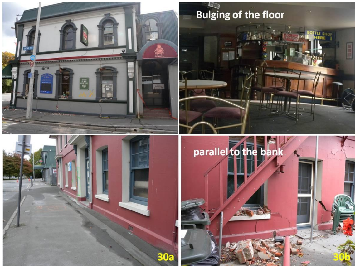
Figure 3.33. Building at Colombo St and Oxford Terrace (B30).
