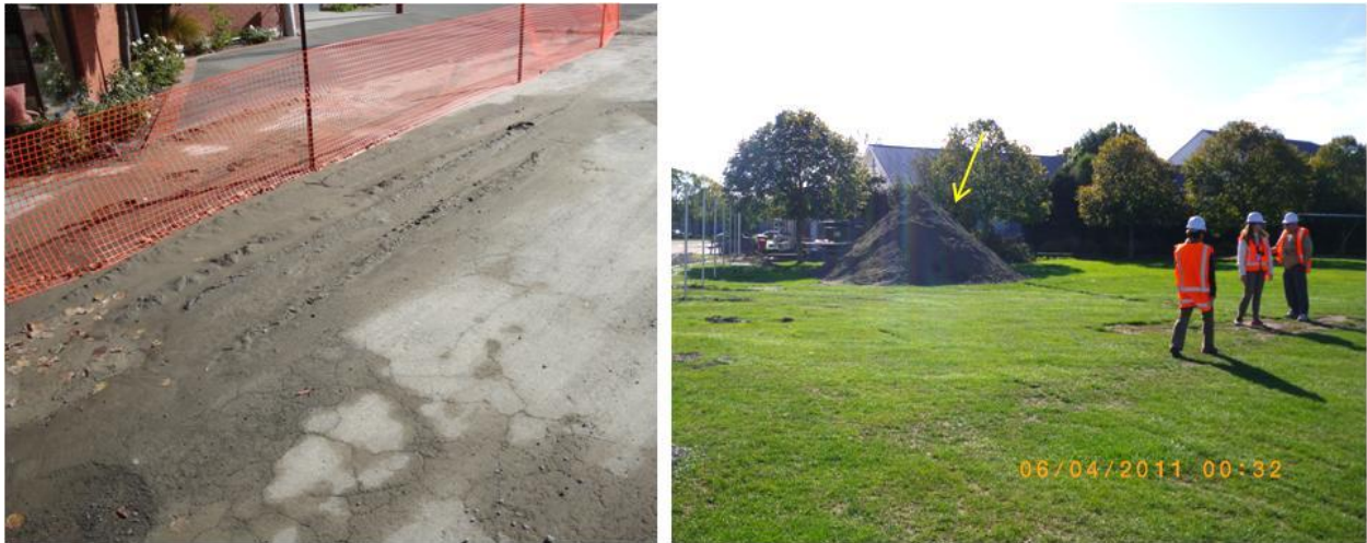
Figure 2.24. Liquefaction in front of Christchurch Cathedral College (right). Ejected sand from the open space next to CCCC station accumulated in a pile (right).
