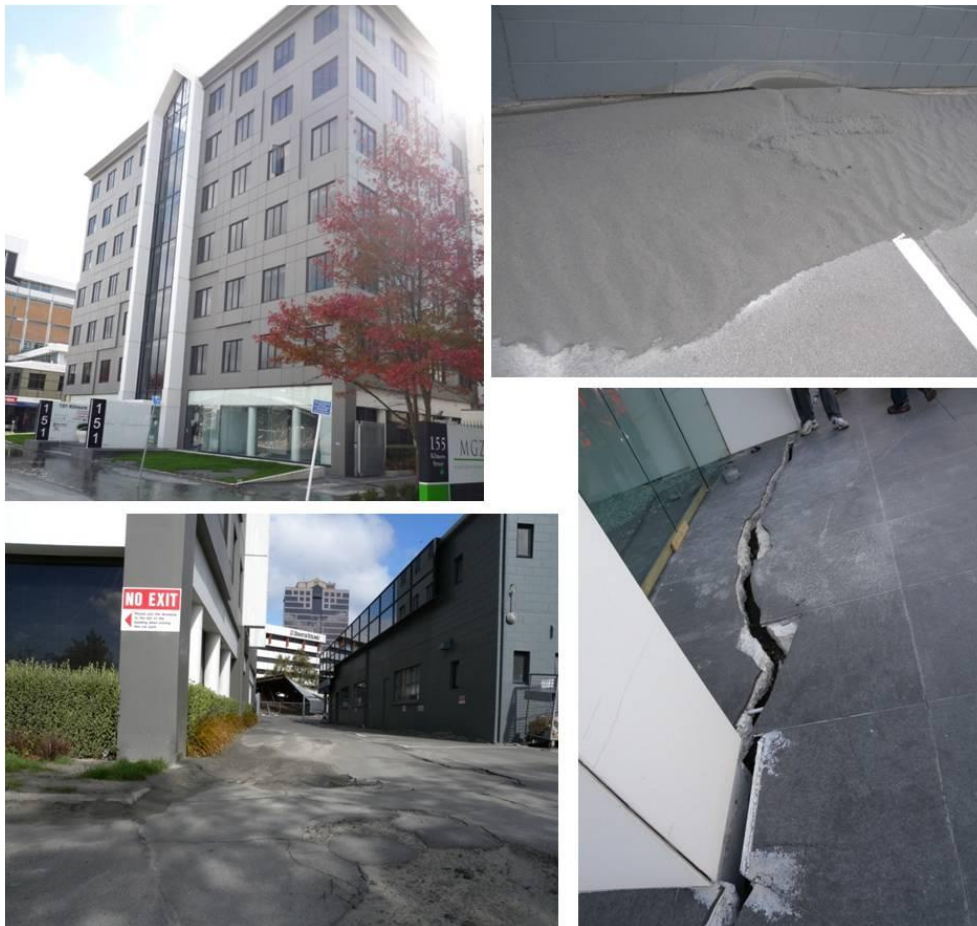
Figure 3.36. A modern RC building at Kilmore Street with raft foundation.
