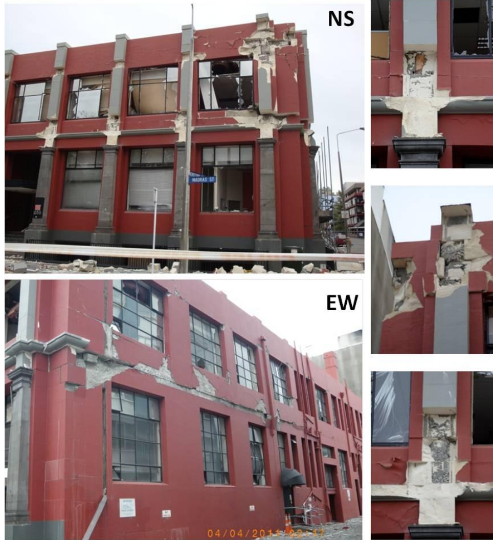
Figure 3.10. Building at Hereford and Madras Streets.
