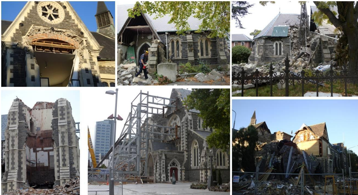
Figure 3.20. Several historical masonry buildings, including the Cathedral, with significant damage.
