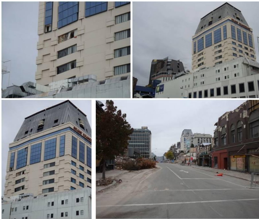
Figure 3.23. Views of the Hotel Grand Chancellor.
