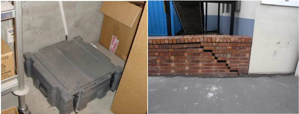
Figure 2.16. Seismograph placed on the ground floor (left). Shear crack in a wall adjacent to CHHC seismic station building due to liquefaction-induced differential settlement and possible heaving (right).
