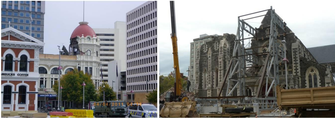
Figure 3.18. Collapse of dome and view of the heavily damaged and partially collapsed Cathedral.
