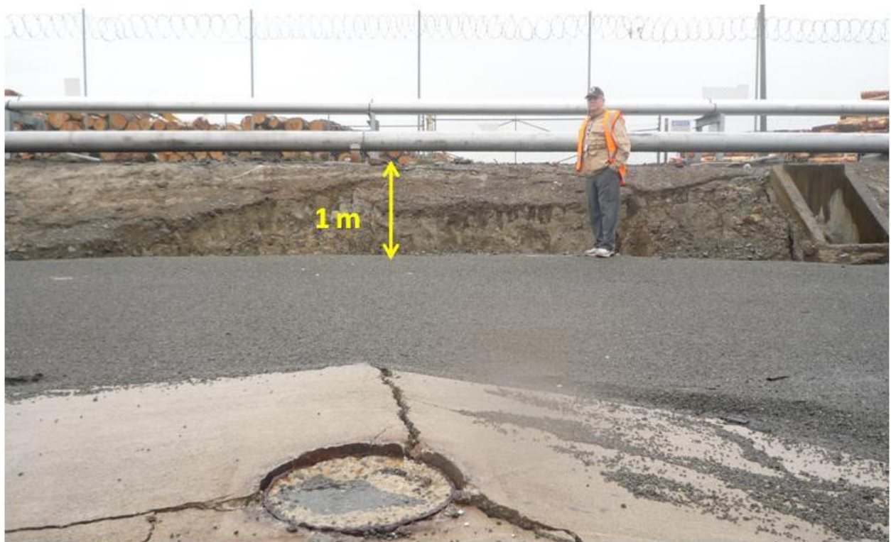
Figure 5.24. Settlement of the backfill in the order of 1 m (site W3 in the map of Figure 5.6).
