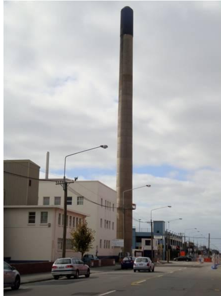
Figure 3.38. A tall RC chimney next to the CHHC recorder (B34).
