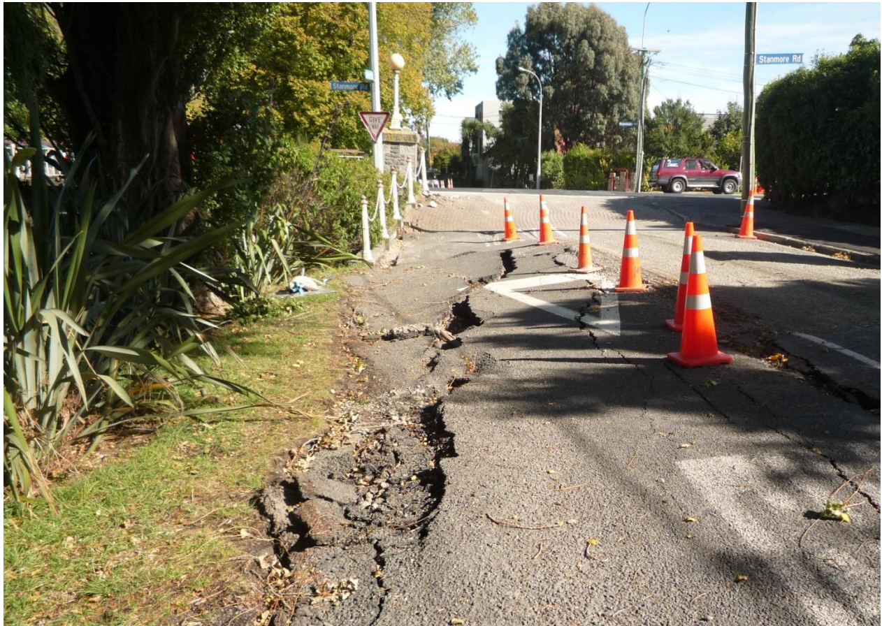
Figure 4.12. Stanmore Bridge (B2 on map of Figure 4.1). Large cracks in the asphalt due to significant lateral spreading in the free field (away from the bridge). The cracks tend to decrease towards the bridge, as the axial stiffness of the deck combined with the bending stiffness of piles limited the lateral ground deformation.
