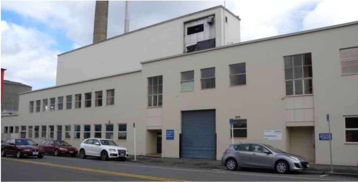
Figure 2.14. 2-storey building at 235 Antigua Street, accommodating CHHC seismic station.
