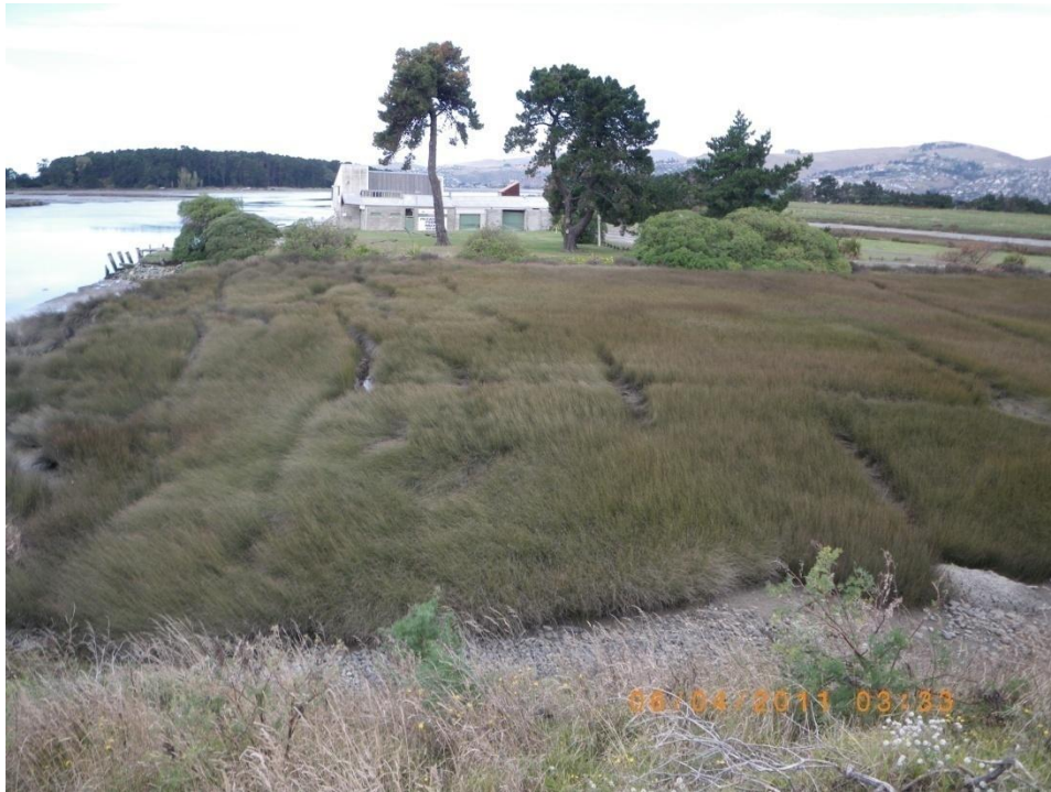
Figure 4.32. South Bridge Road Bridge (B8 on map of Figure 4.1) after Christchurch earthquake. Large lateral spreading cracks in the ground parallel to the coast and adjacent to the abutments extending at a great distance inland.
