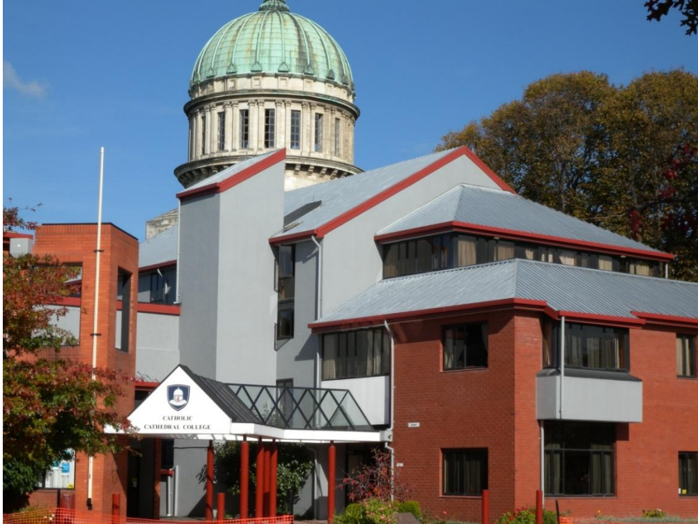
Figure 2.22. Christchurch Cathedral College building accommodating CCCC seismic station.
