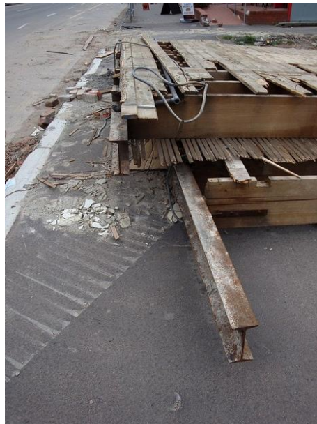
Figure 3.5. A composite slab found at Manchester Street.
